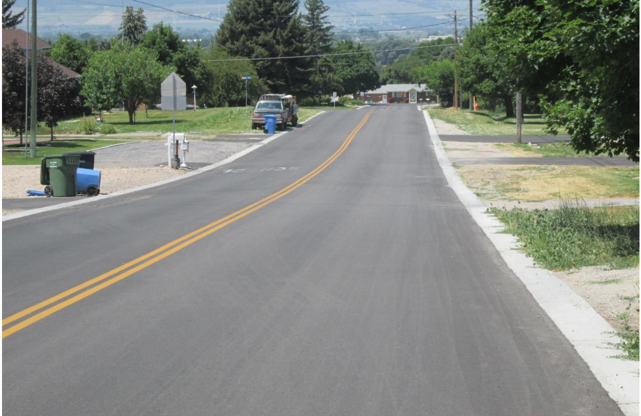
Photo 5. Excellent Condition – 400 S from Main Street to 100 W (RSL = 20 years)
