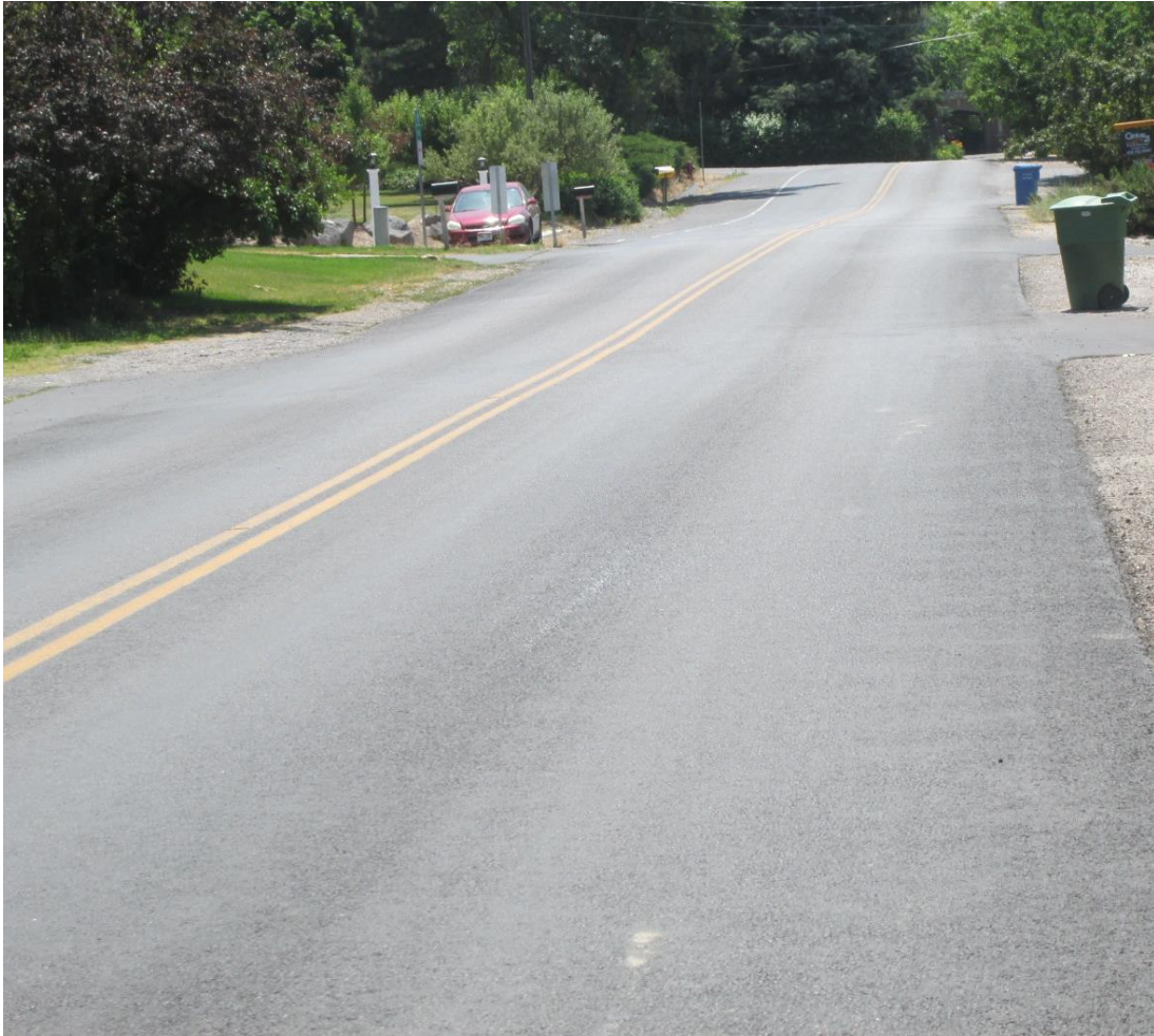
Photo 4. Very Good Condition – 300 E from 300 S to 400 S (RSL = 14 years)
