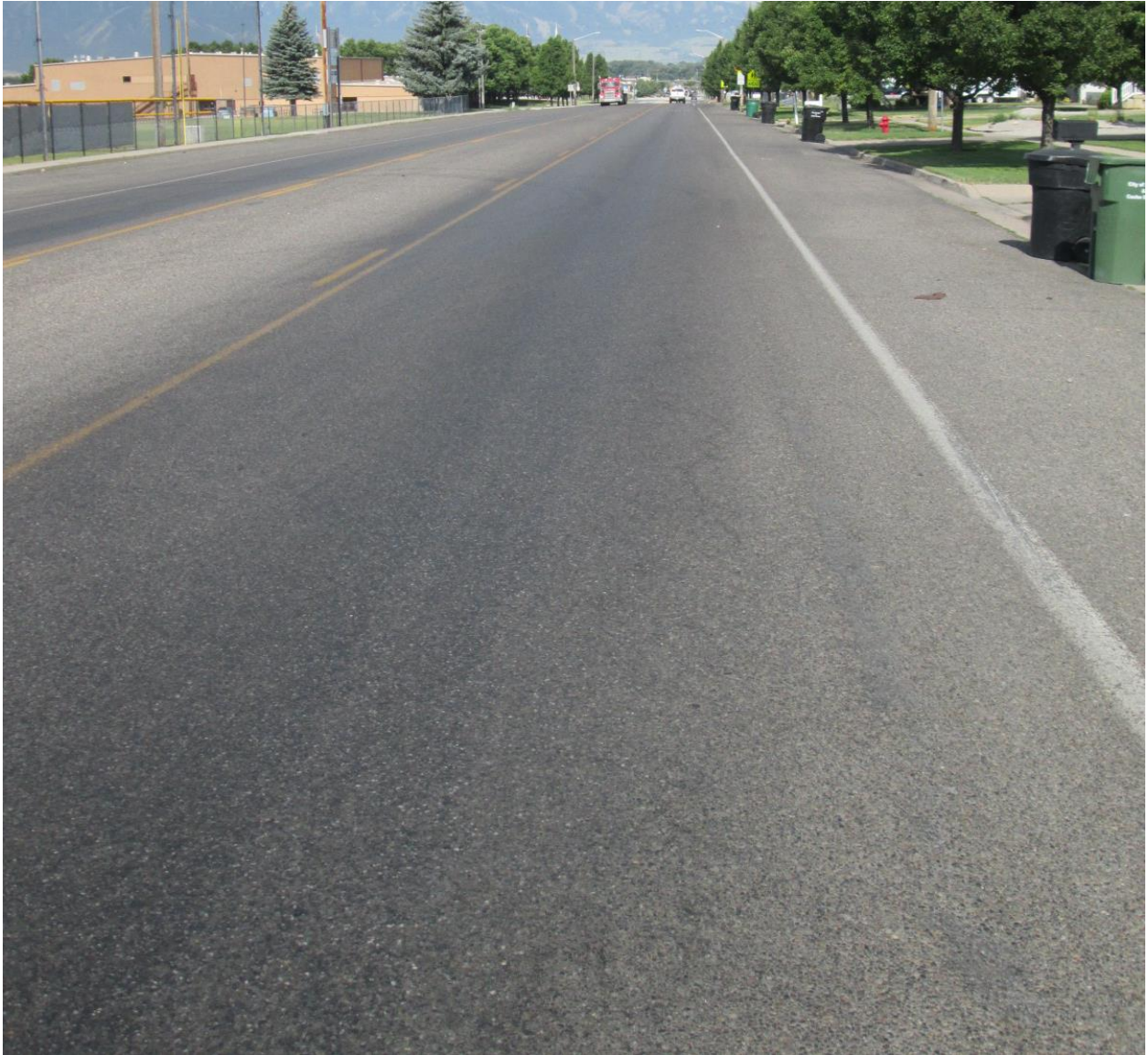
Photo 3. Good Condition – 100 N from 200 W to 300 W (RSL = 10 years)
